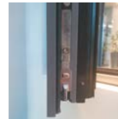
Bottom locking point on sash
