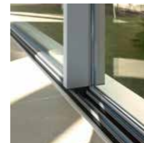
Detail of the central overlap of two panes, showing lower frame flush with the outer and inner pavement. The depth of the pane upright depends on the pressure it must support so that the glass does not exceed its stress threshold.
