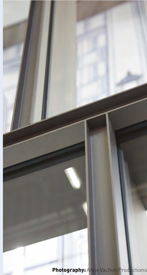
Asymmetrical frame and U type cap
