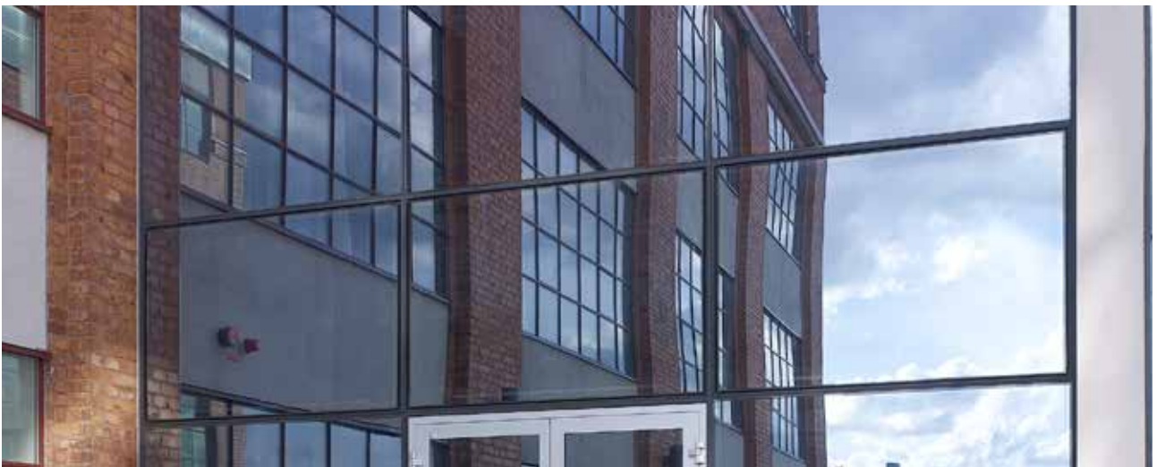
Facade window 4074, closed position.
