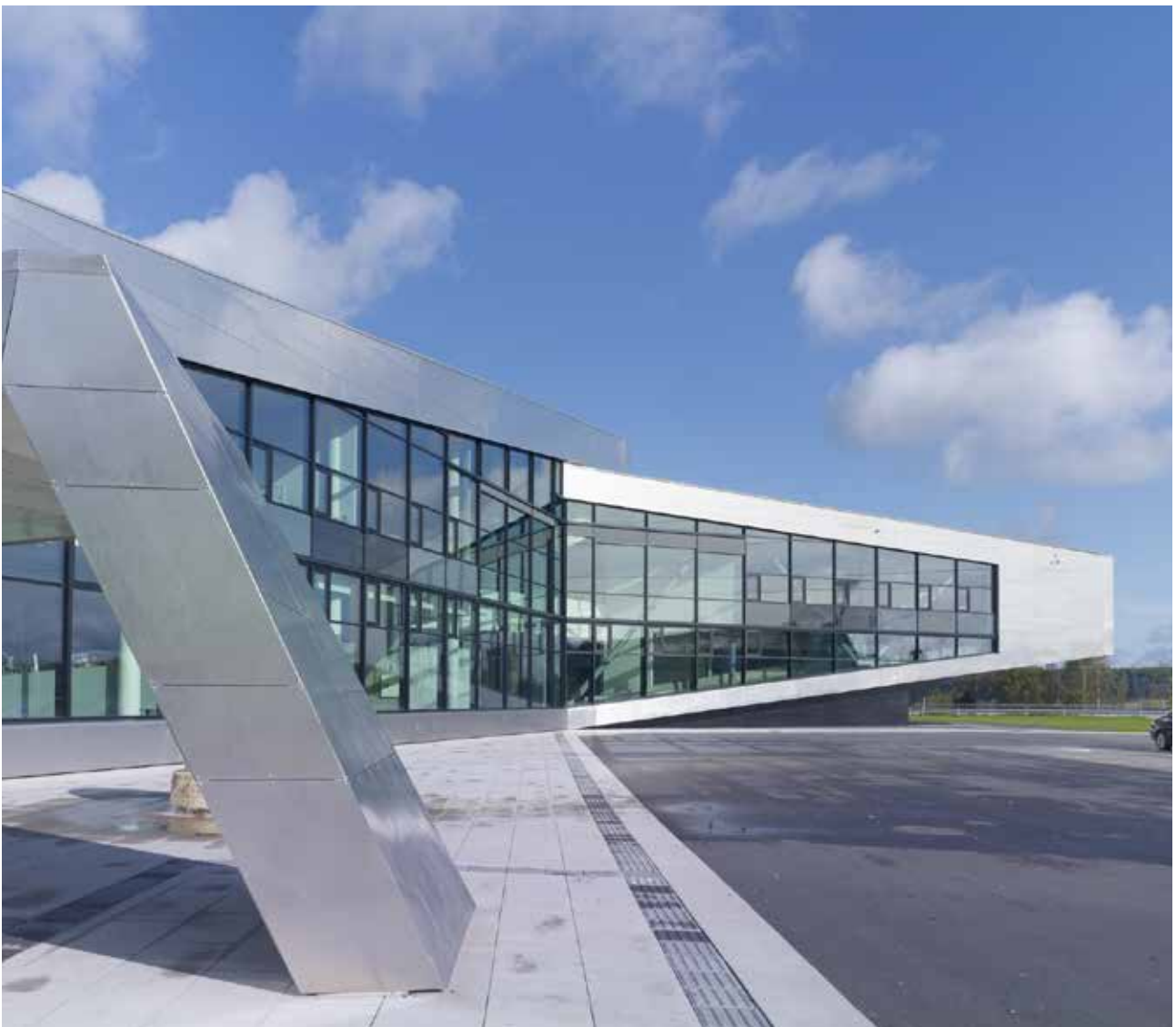
Sapa 4150 SX at the Science and Innovation Centre in Sarpsborg, Norway.
